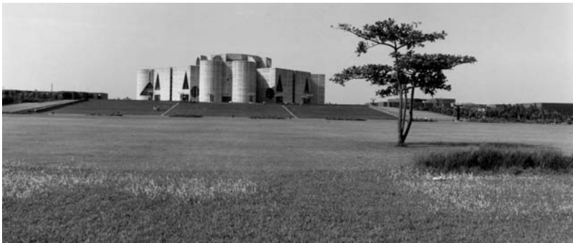
Figure 3.15. Isolating the capitol: Dhaka, Bangladesh. The capitol complex for Bangladesh occupies its own district, set well apart from the bustle of the city.
