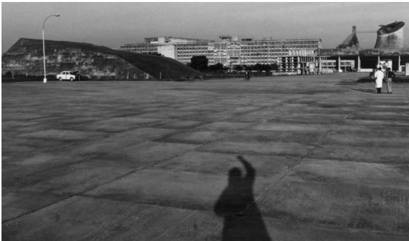
Figure 3.11. Capitol Complex, Chandigarh. Le Corbusier’s design for the capitol complex at Chandigarh is a complex system of plazas and framed views, but the result is a pedestrian-resistant expanse of paving. The sense of isolation is further enhanced by the artificial mound (on the left), constructed to block the view of the rest of the city.
