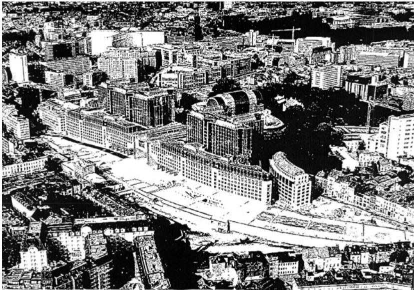
Figure 17.7. Aerial view of the European Parliament complex in Brussels. The oval hemicycle building with the half-barrel shaped cupola is the Paul-Henri Spaak building. The administrative offices in the Altiero Spinelli Building are alongside the covered railway tracks. The Gare du Luxembourg is on the axis of the Parliament, with the neoclassic Place du Luxembourg beyond. In the background are the Council building Justus Lipsius and the Berlaymont, headquarters of the Commission, under reconstruction.
