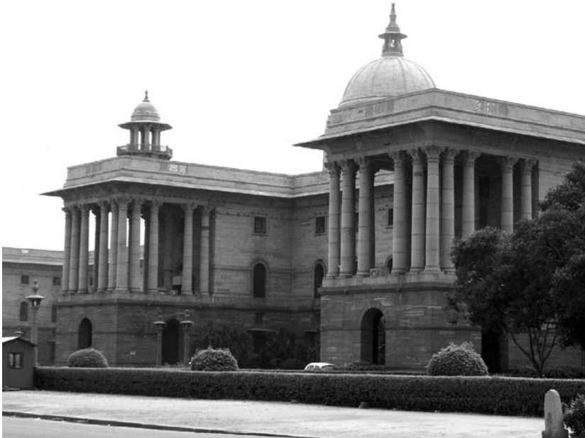
Figure 13.3. The south Secretariat Building designed by Herbert Baker.
