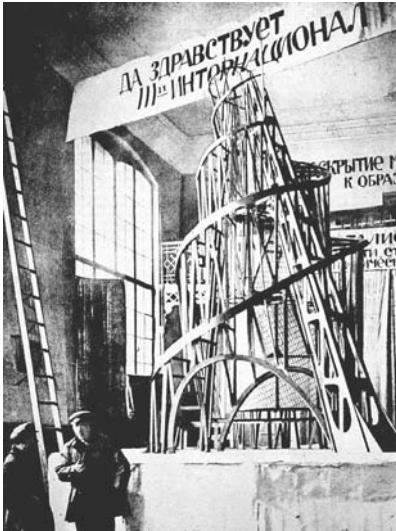
Figure 5.4. Monument to the Third Internationale by V. Tatlin, in Soviet abstractionist avant-garde style, was also designed as a functional building proposal with revolving internal volumes suspended on cables, in studio, Petrograd (Petersburg), 1919.
